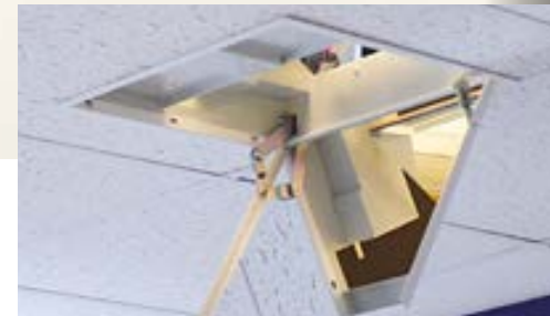
Mirror mount installed in false ceiling
